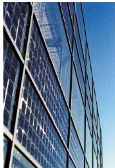
Figure 1: Building presenting photovoltaic solar panels in its facade
